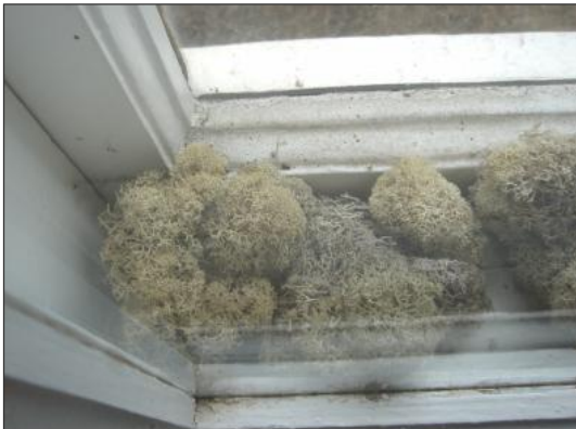
Historically, star-tipped reindeer lichen was put between windows to absorb any moisture and prevent water from soaking into the wood
